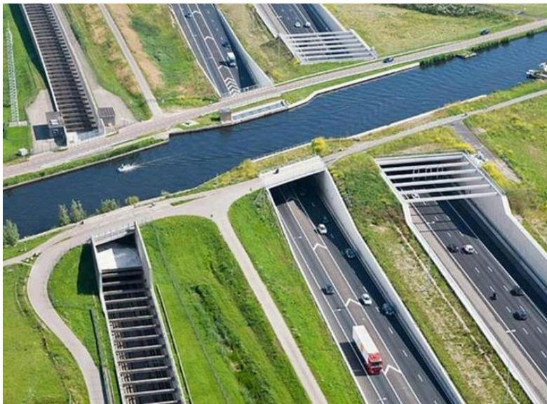
6.3 – Aqueduct Ringvaart over the A4 Highway, Haarlemmermeer, The Netherlands (2006).
