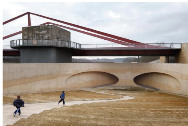
5.15 – Open Call 0229 bridge in Vroenhoven (Source: FGA, 2019 © Stijn Bollaert)
